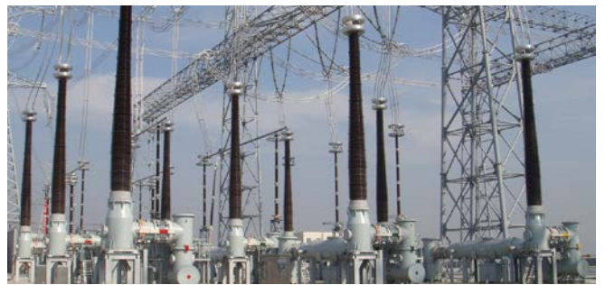
Ultra-high voltage gas insulated switchgear (UHV GIS)
