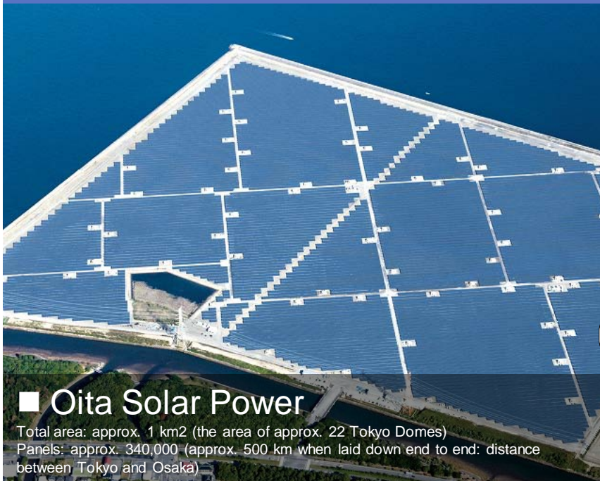
Japan's largest class mega-solar systems (82 MW-class)
