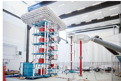
High Voltage and High Power Testing
