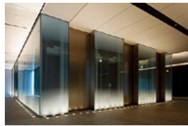
Elevators* supplied to AKIHABARA UDX
