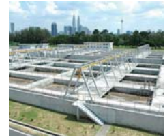
Sewage treatment plant built by Hitachi Plant Technologies, Ltd. in Malaysia
