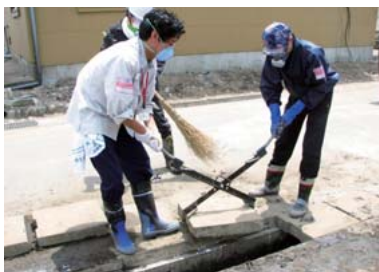
Clearing away the sand piled up on roads by the tsunami
