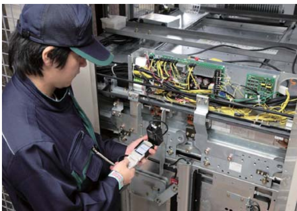
Maintaining an elevator control board
