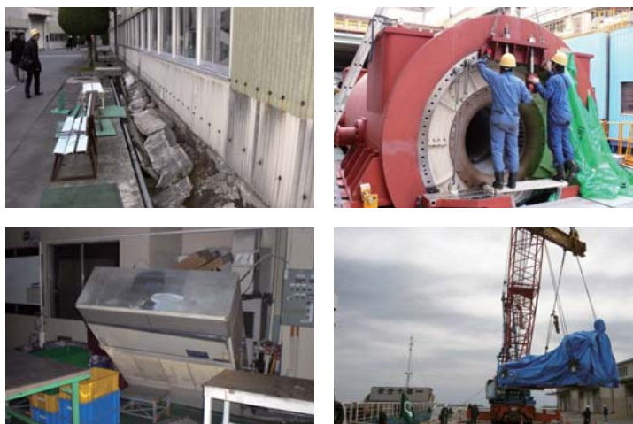
Cracked road at Hitachi Works (top left) Toppled air conditioner inside the plant (bottom left) Power generation machinery assembly resumes (top right) First post-disaster gas turbine shipped from Hitachi Port (bottom right)
