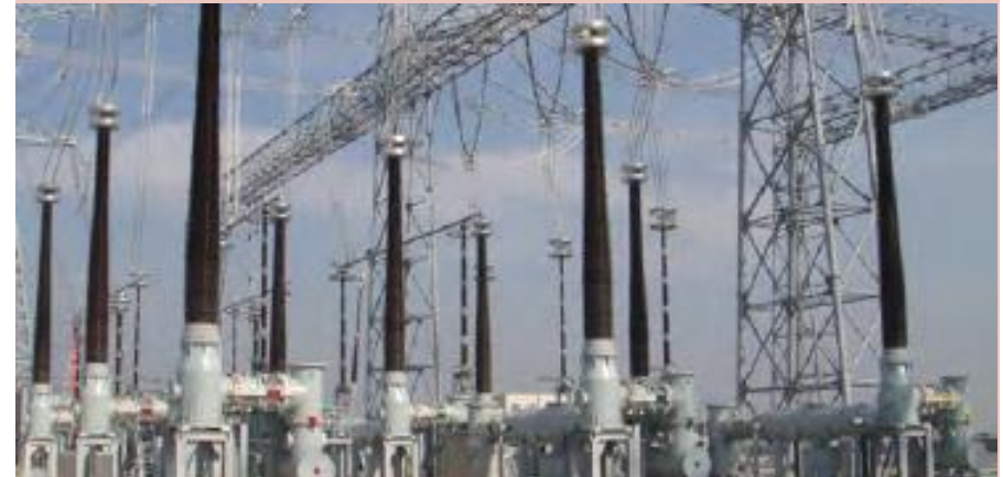
Ultra high voltage (UHV) gas-insulated switchgear
