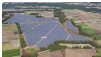
Completion of Ichigo Showa Village Ogose ECO Power Plant (October 2017)
